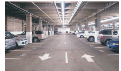
Basement Parking Area
