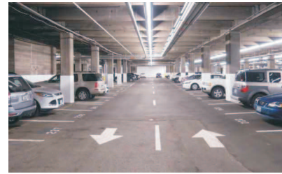
Basement Parking Area
