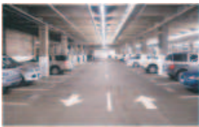
Basement Parking Area
